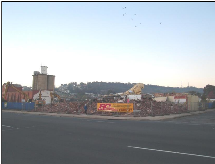
Left: Red Lion Hotel demolished. 15 th May 2012
