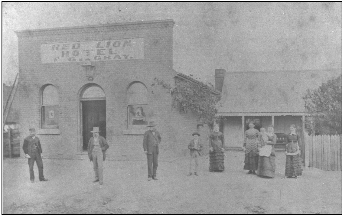
Above: The Red Lion hotel & residential cottage - pre 1880. Photo courtesy Graham & Margo Trimnel
