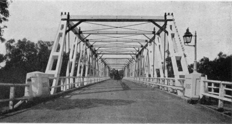
Deck of Hampden Bridge.
