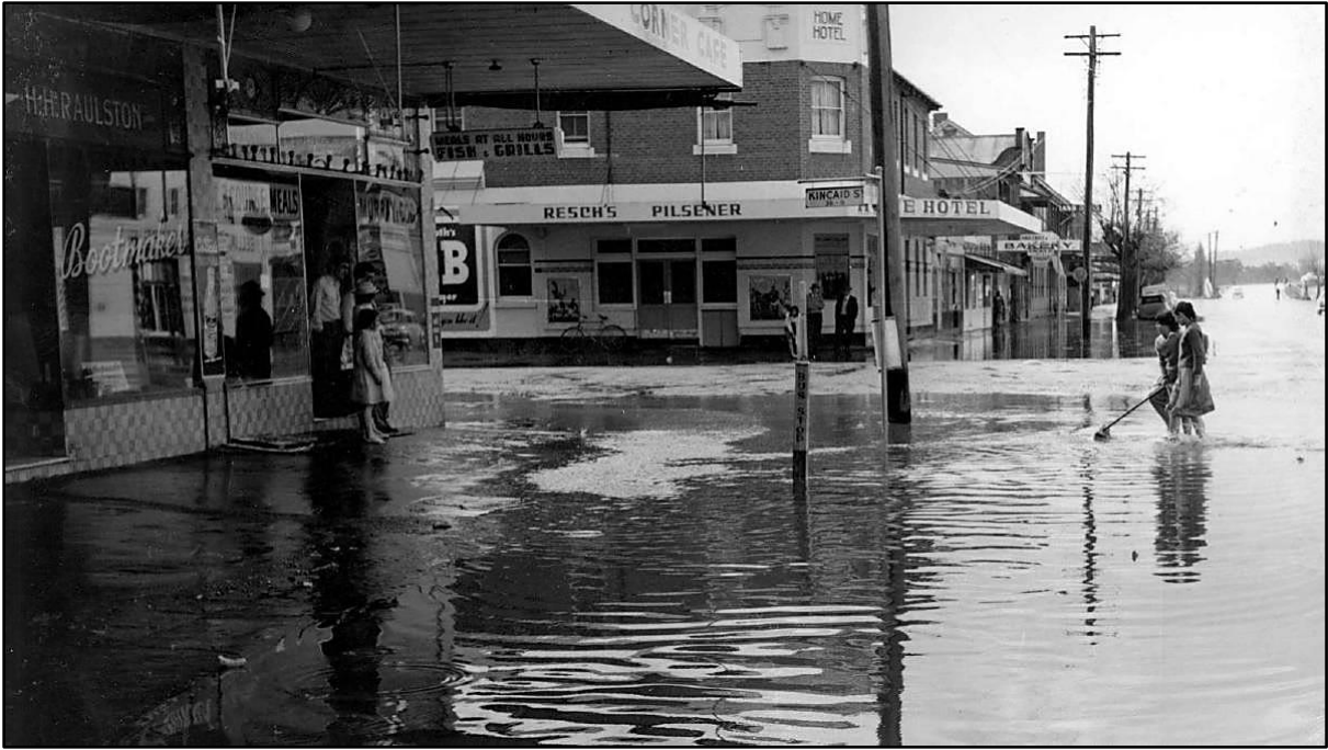
Above: Crown Corner – Corner Café to the left and Home hotel in centre, in period of flood.
