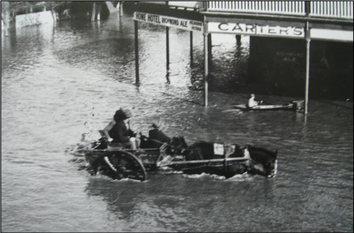
Above: A serious flood in 1932.
