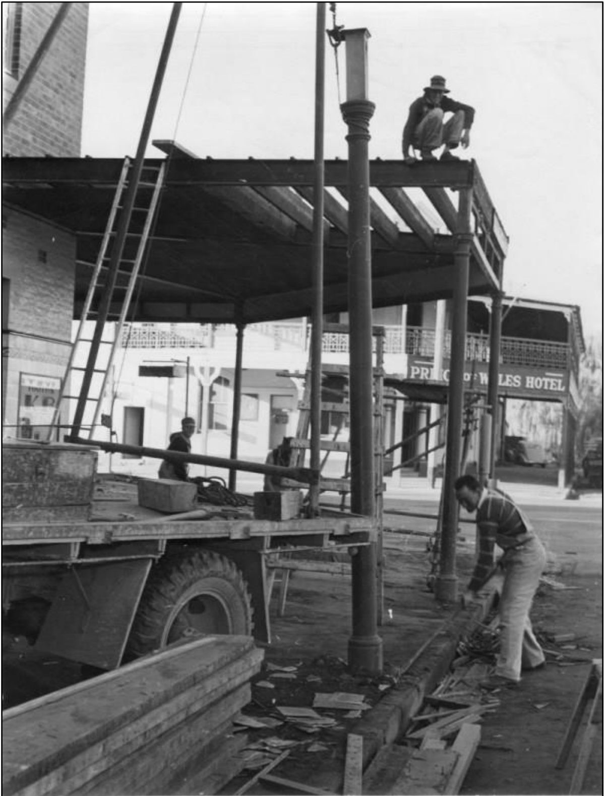
Above: Removing the verandah of the Home hotel, with the Prince of Wales hotel in the background. Photo courtesy Daily Advertiser. Tom Lennon Collection. RW1574/596.
