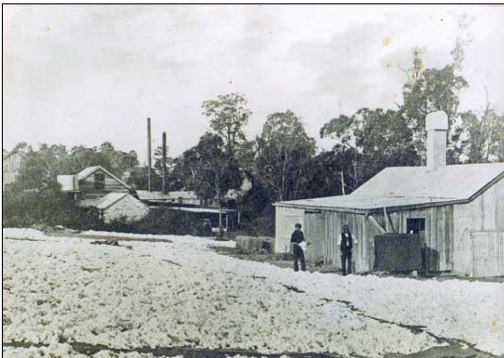
Above: Scoured wool spread out to dry in the sun. Photo courtesy the Chermside & District Historical Society. This procedure would have been practised at each of the Wagga Wagga scouring works, it being an essential component of the scouring process.
