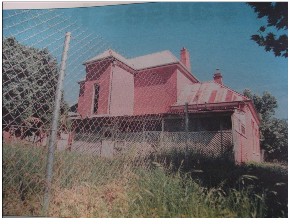
Above: A fence around the derelict site
