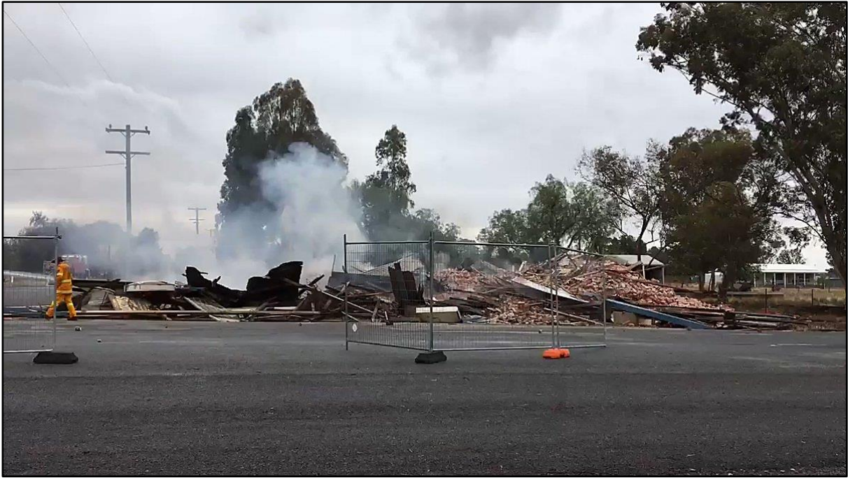
Above: Completely demolished. Now just a pile of rubble. Courtesy Twipu. Marguerite McKinnon. 2018.
