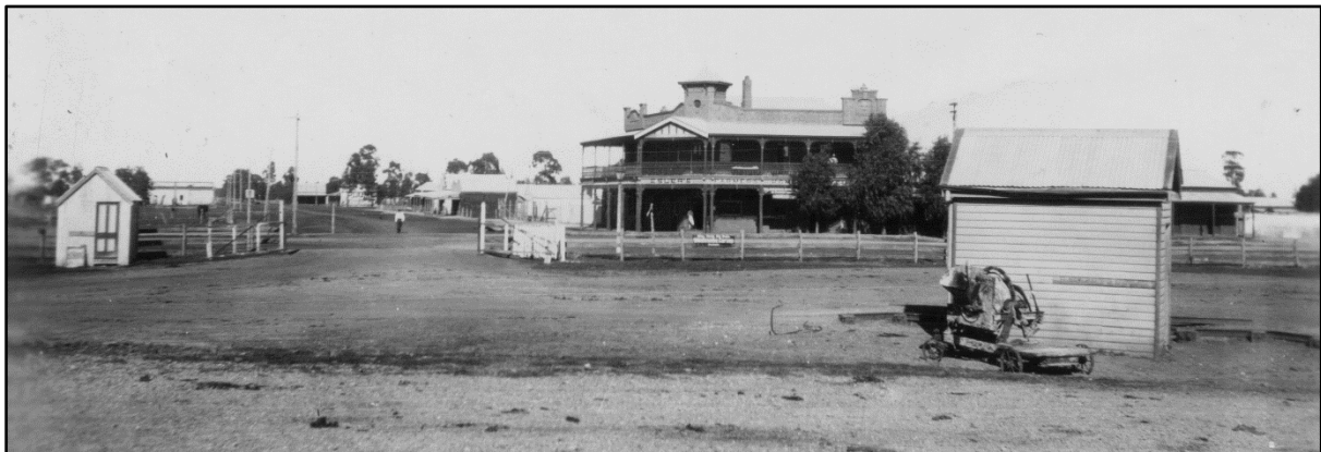
Above: Looking at the Farmer's Home hotel across the railway line.
