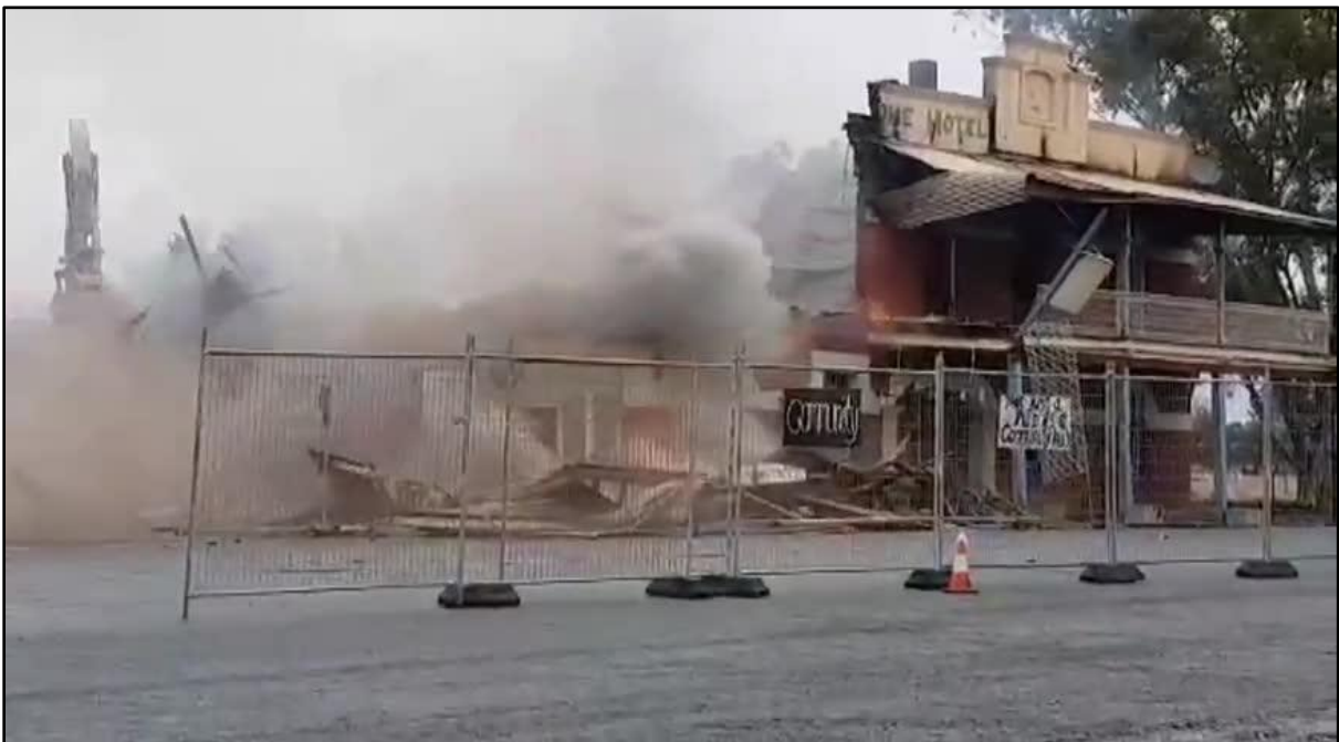
Above: Being demolished in 2018. Courtesy PRIME7 News.
