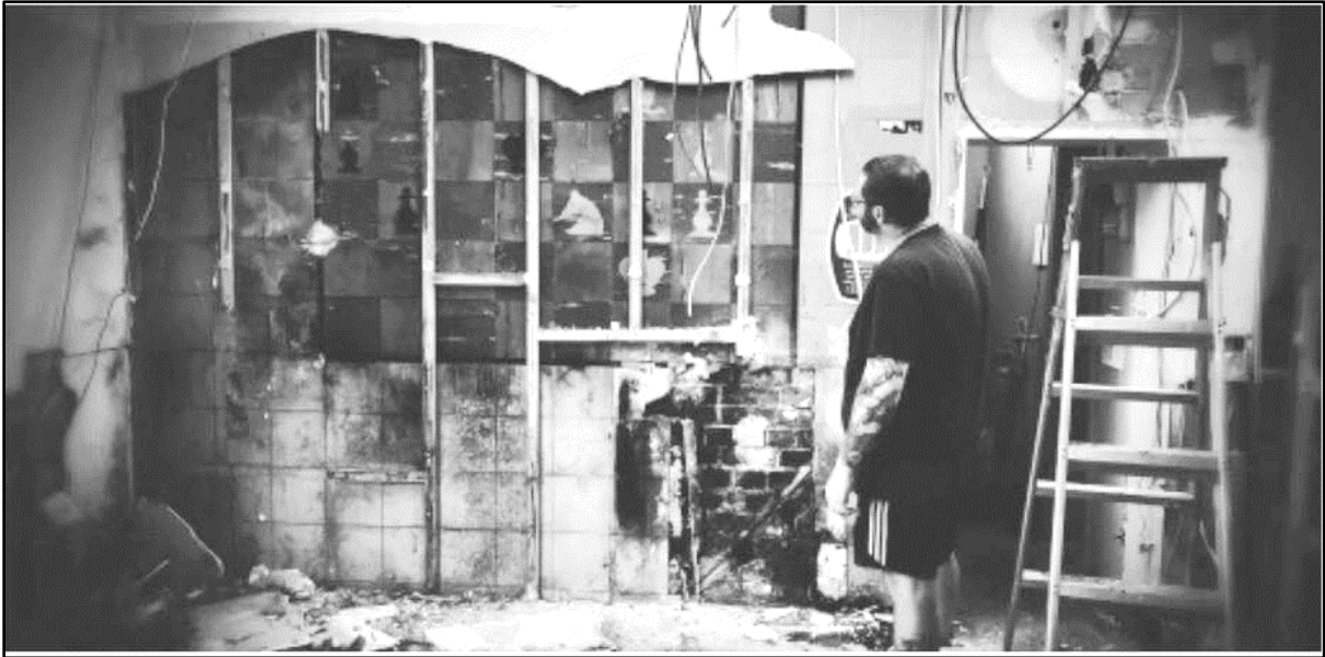
Above: The hidden chess wall revealed during renovations in April 2018. Courtesy Lost Wagga Wagga.
