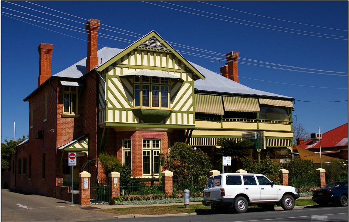
Above: The Manor in 2012. The large trees that once stood at the front of the building are now gone.
