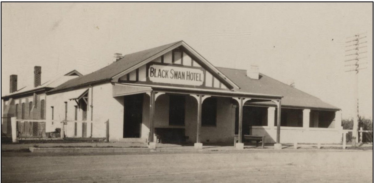
Above: The Black Swan hotel in 1928. Note additions to the rear of the hotel and the new facade. Courtesy Tooth & Co. records. Yellow Cards. Noel Butlin Archives. ANU, Canberra.
