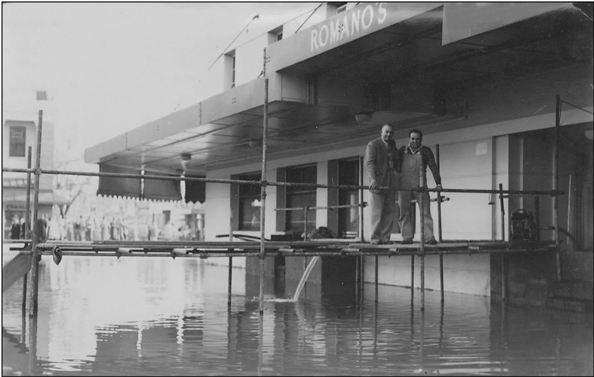
Above: Another flood photo. Pumping water out of the hotel – presumably from the cellars. Courtesy Museum of the Riverina [BGS2013_1016b].
