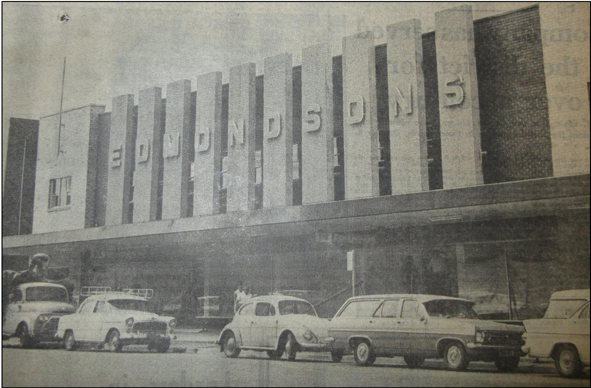
Above: The new $1 million Edmonson's Store in October 1969. 145
