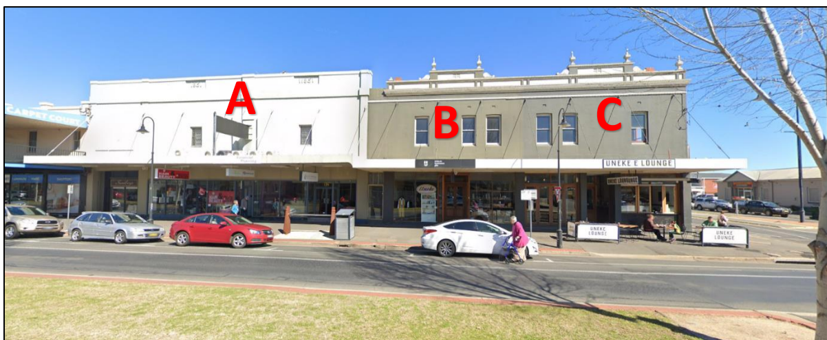
Above: The site in 2020 [Allotment 8, frontage to Fitzmaurice Steet]. Courtesy Google Maps.
