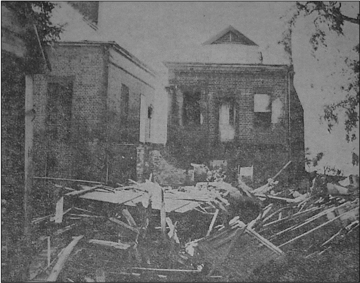
Above: A photo of the demolition works in 1966. Courtesy Daily Advertiser.
