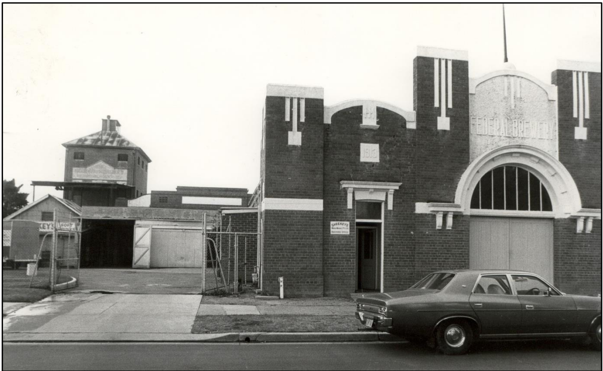
Above: The Federal Brewery in April 1978.
