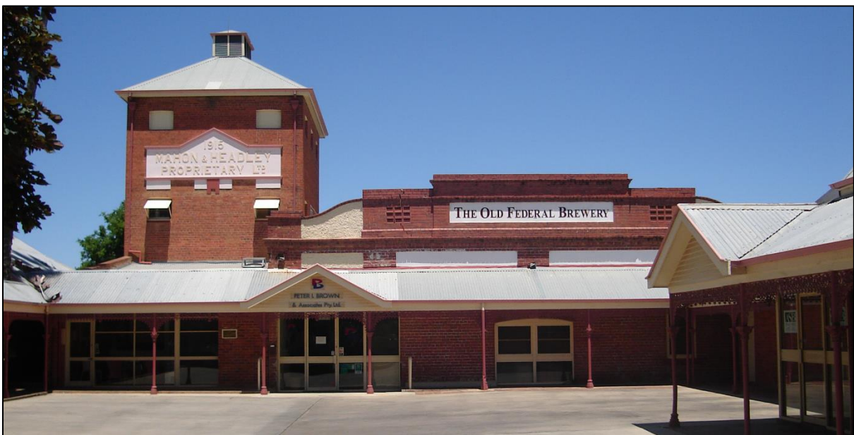
Above: The old brewery buildings in 2010.
