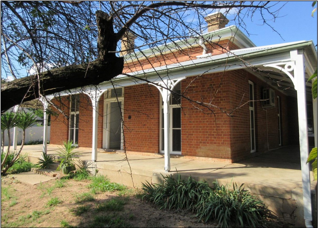
Above: Mount Austin homestead in 2021 – viewed from south west corner.
