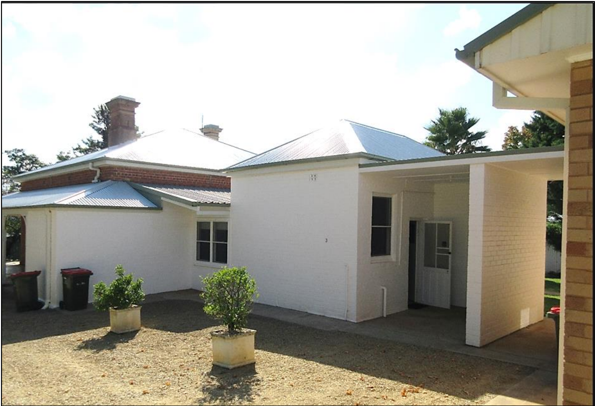
Above: The Mount Austin homestead, viewed from the southern side, at the rear, in 2021. From left to right can be seen the main homestead building, the old kitchen and thirdly the rear of the two flats to the north. The addition of a connecting piece can be seen between the main building and the old kitchen. An alcove with roof has been added to the old kitchen.
