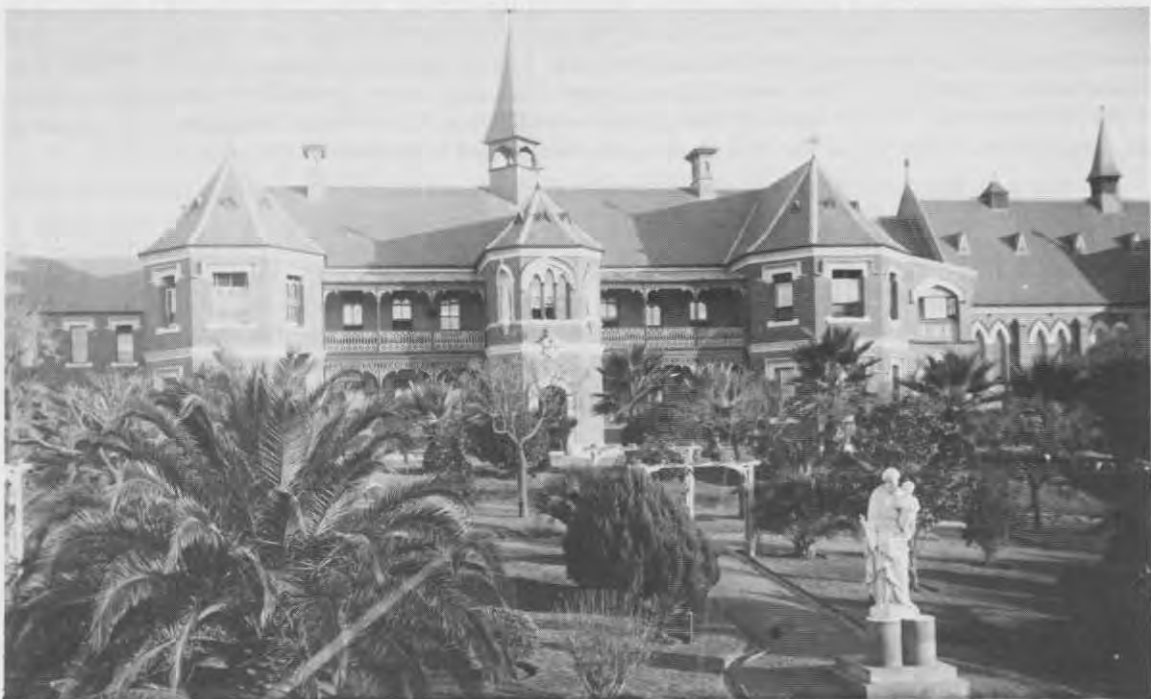
Mount Erin Convent showing portion of Boarding School and Chapel
