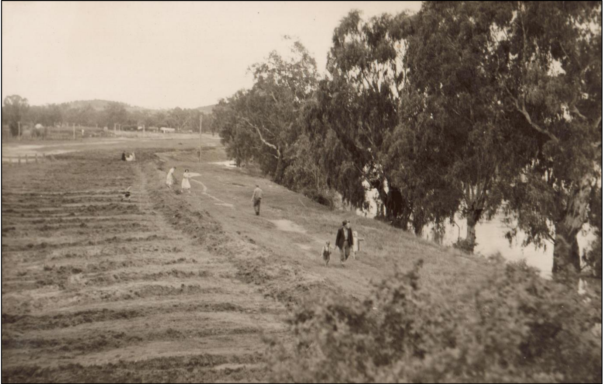
Above: Temporary levee bank works in 1950. Courtesy Museum of the Riverina. [BGS.2004/268bc]
