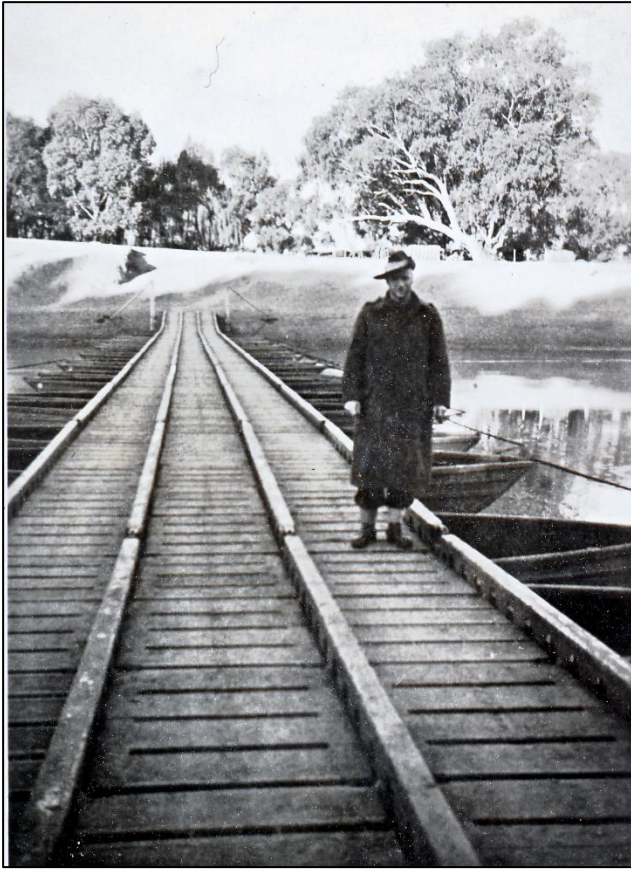
Above & Below: More photos of the pontoon bridges built by the Royal Australian Engineers.
