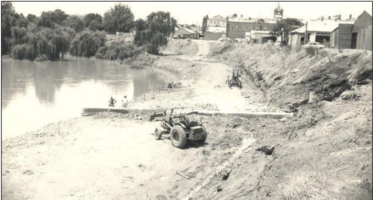
Above: Work on the permanent levee bank in 1960. Courtesy Museum of the Riverina. {RIV.2009/1160a}
