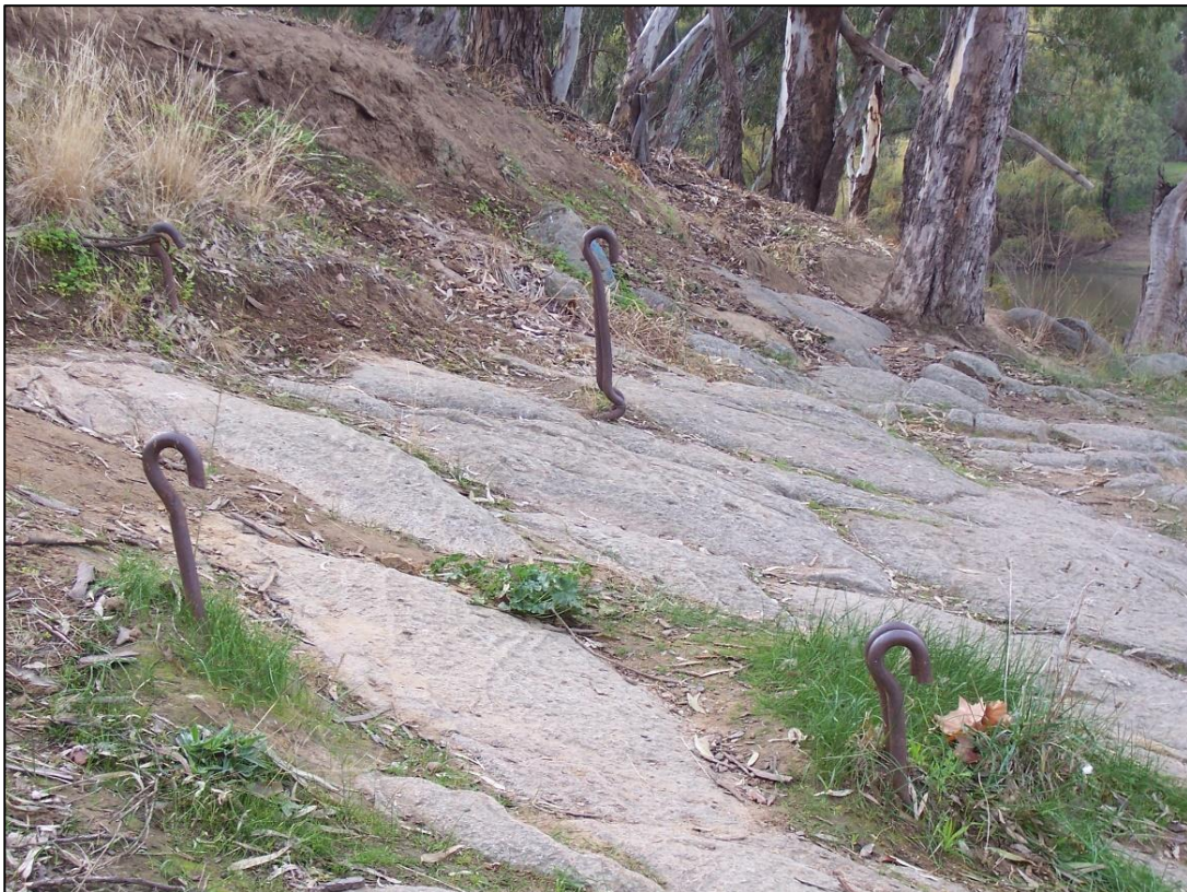
Above: Steel hooks set into stone at The Rocks area [in 2020], believed to have been used by the engineers, in the 1940's, to secure the cables across the river.
