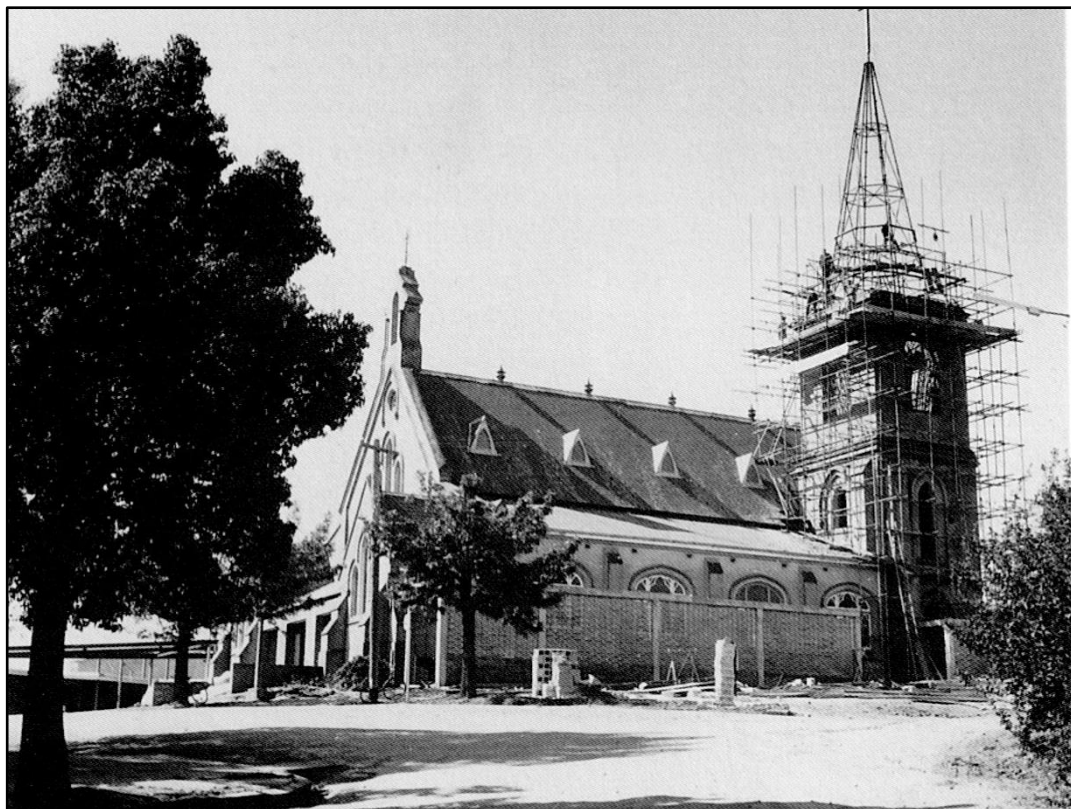
Above: Construction of the new bell tower and spire in 1964-1965. 133
