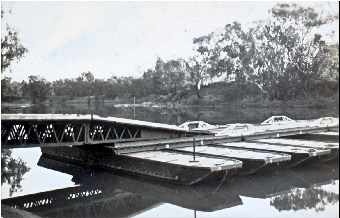
Above: One of the pontoon bridges constructed by the Royal Australian Engineers during WW2.
