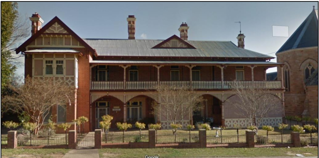
Above: The Catholic Presbytery in 2019. Courtesy Google Earth.
