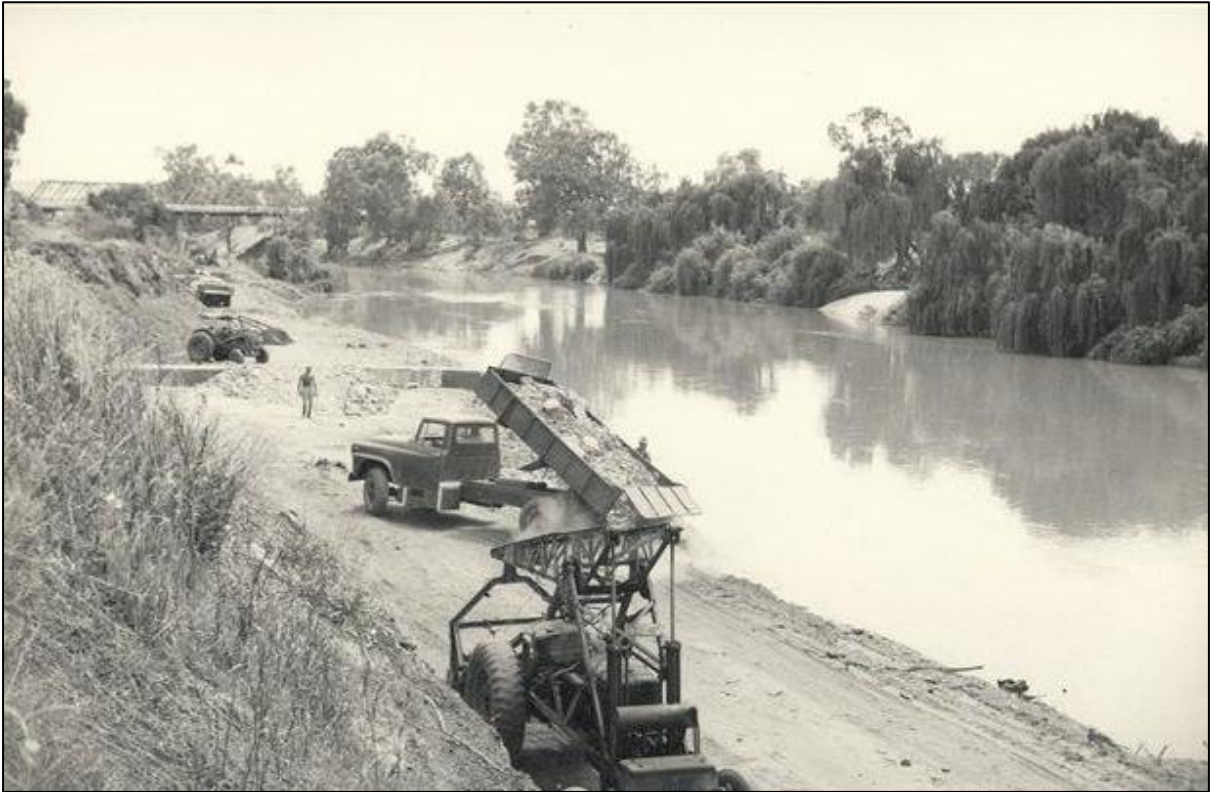
Above and Below: Work on the permanent levee bank in 1960. Courtesy Museum of the Riverina. {RIV.2009/1160b & 1160c}
