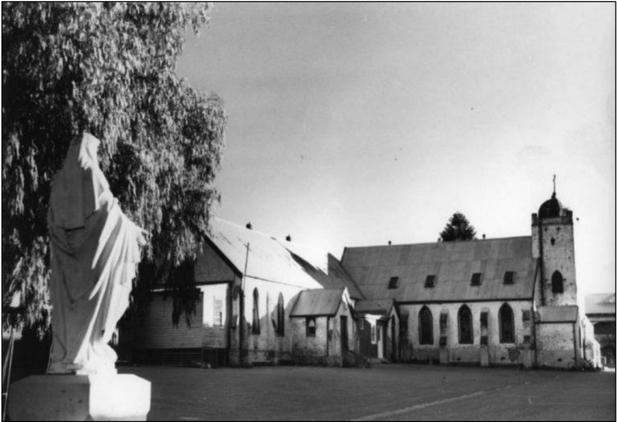
Above: The original St Michael's church building with the 1875 additions [at rear].
