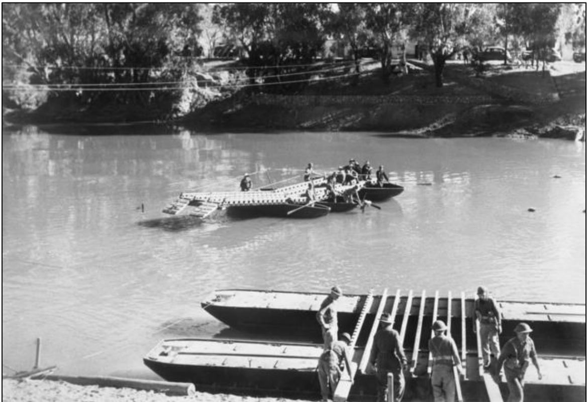
Above: Construction of a pontoon bridge in 1943. Courtesy Australian War Memorial. [052551].
