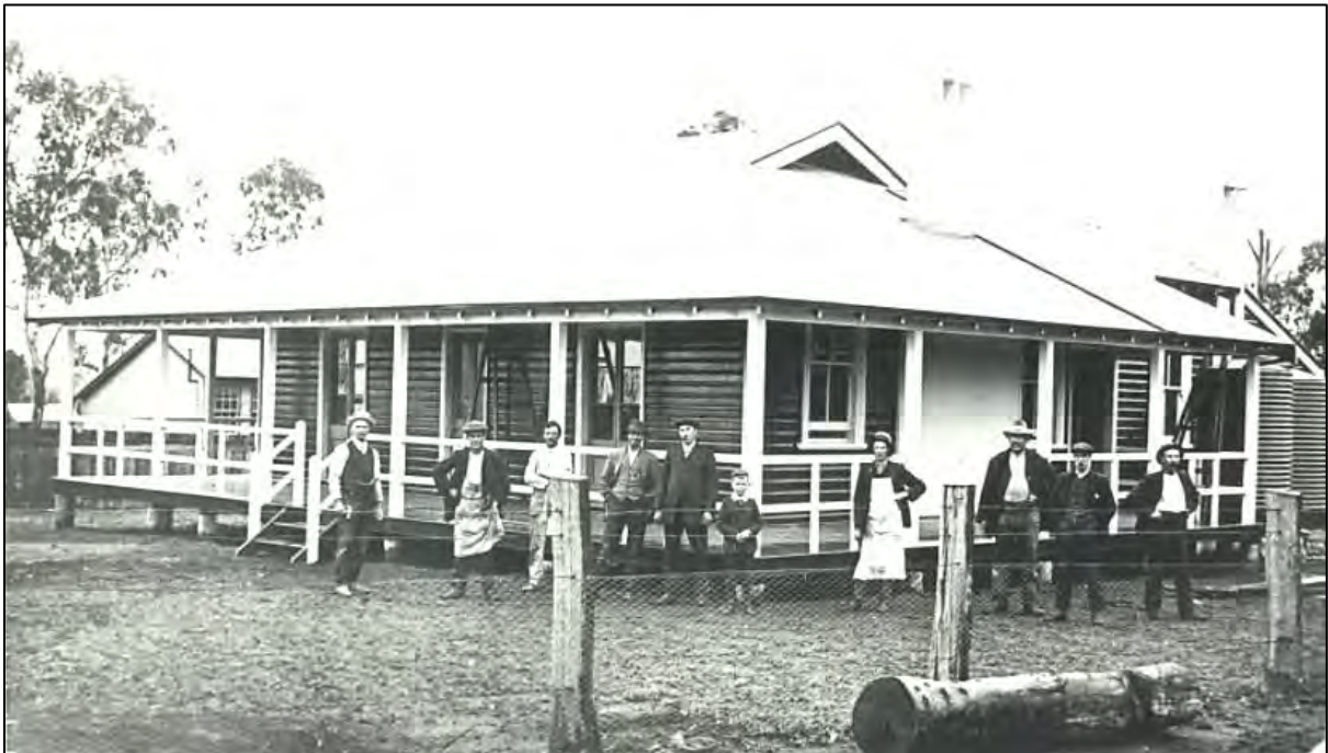
Above: Marrar Public School during construction in 1913. Courtesy NSW State Records. [NRS-15051-1-22-[1181]-1]
