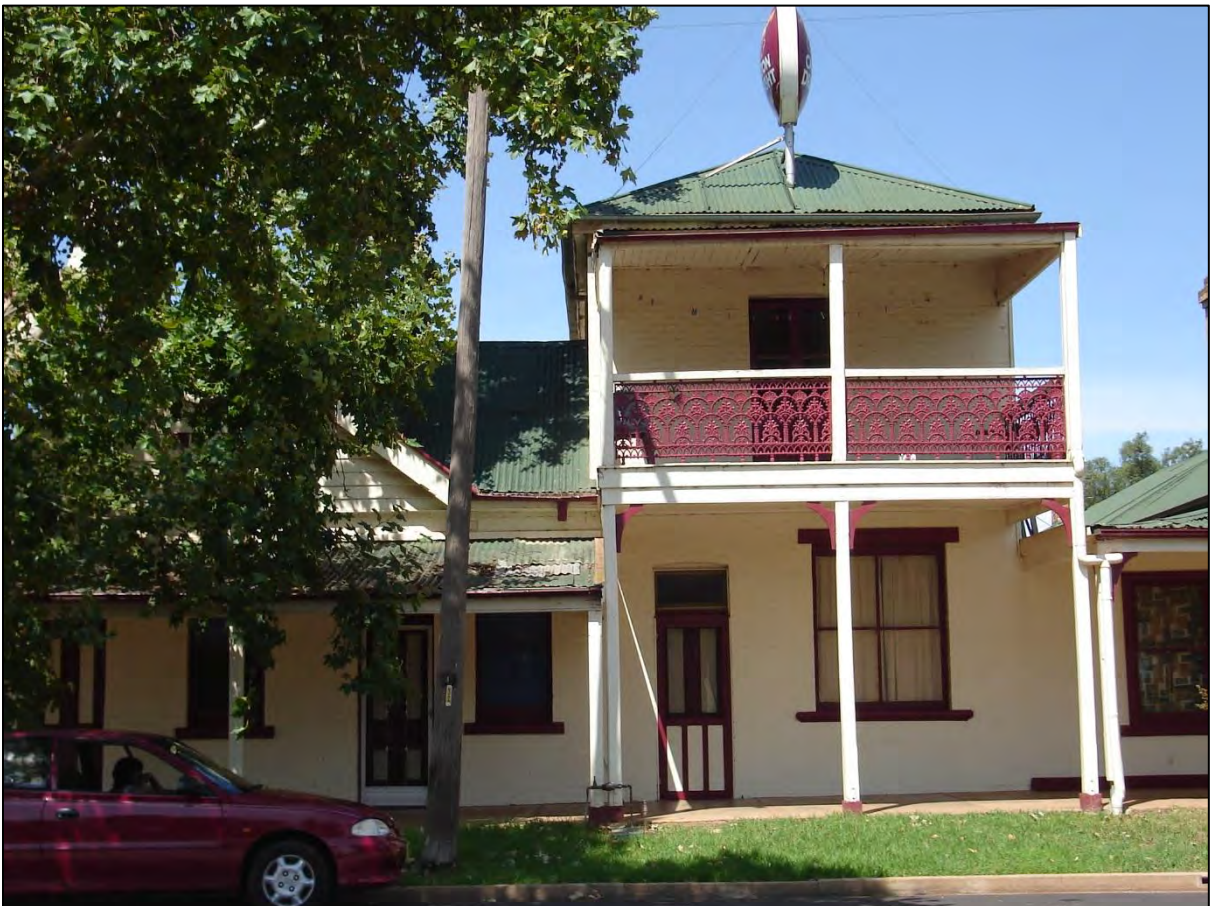
Above: The old two storey building and the adjoining building to the east, in February 2010.
