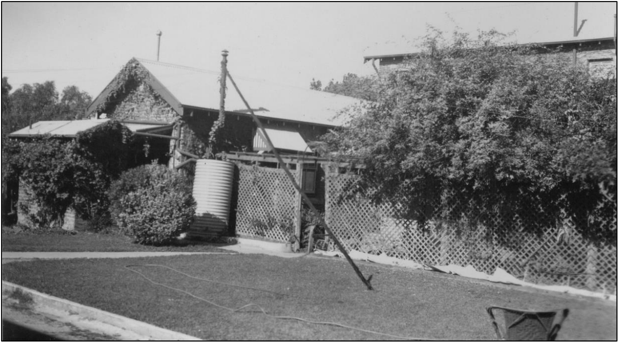
Above: Back of hotel, showing laundry and old water closet [1960's]. Courtesy Tooth & Co. Records. Noel Butlin Archives. ANU, Canberra.
