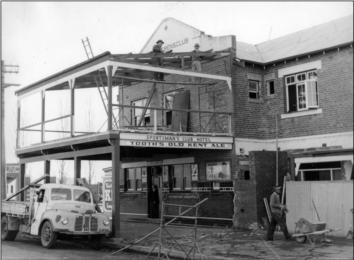
Above: Removal of the veranda. Courtesy CSURA [RW1574-1560]
