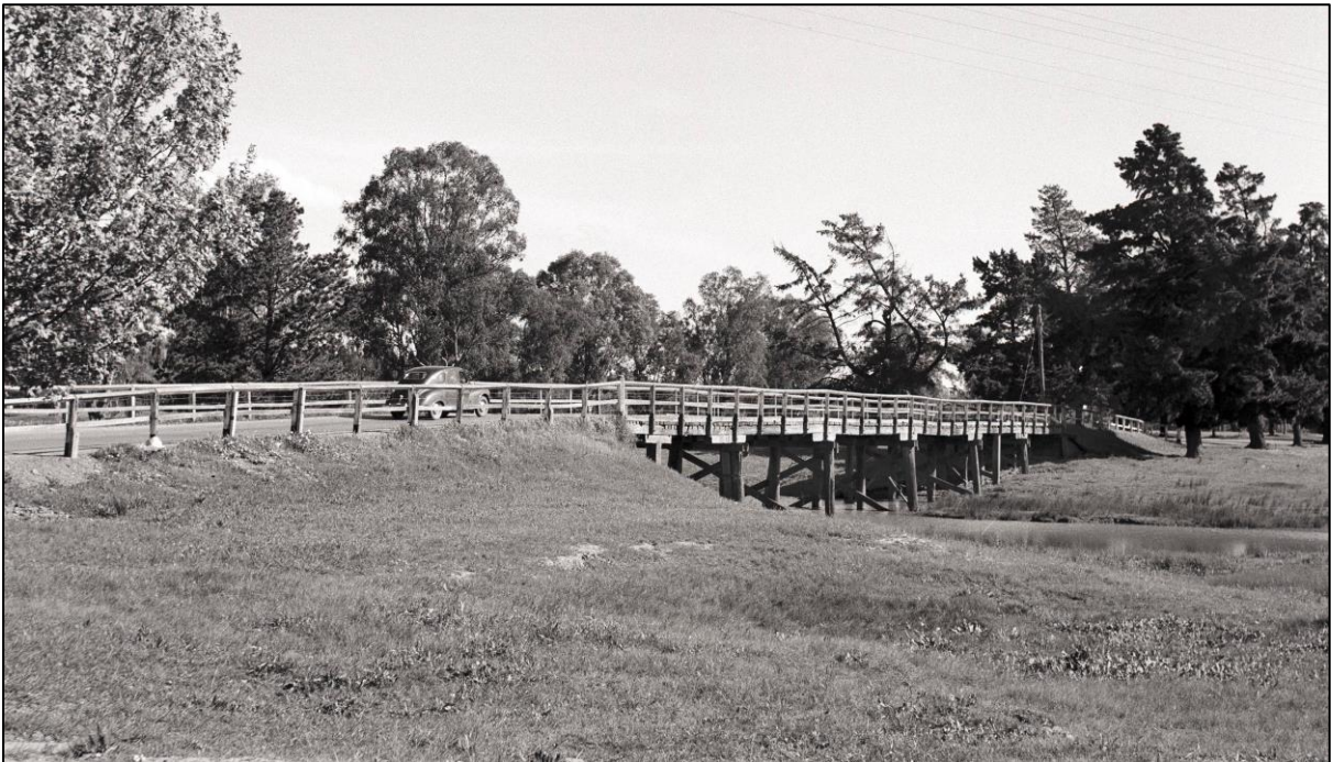
Above: Parken Prgan Bridge in 1952.
