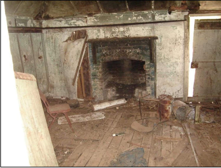
Left: Fireplace inside the old Warri homestead building – in 2014.
