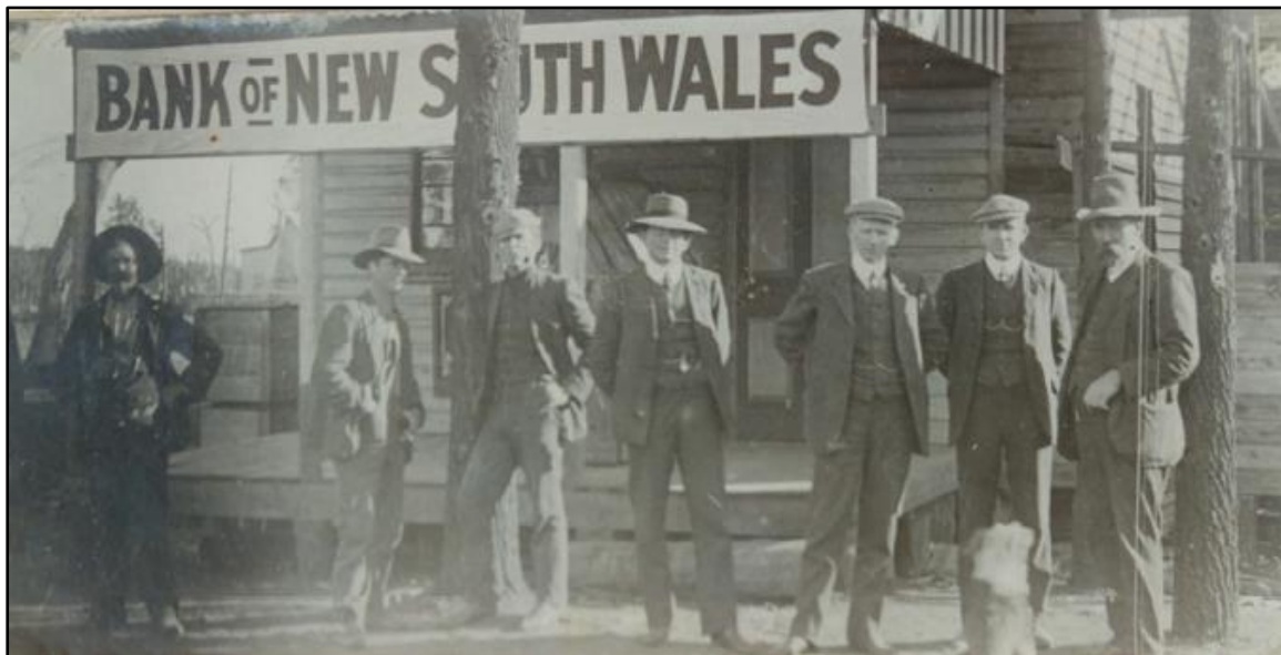
Above: The original Bank of NSW building in Mirrool Street (to the south of the London hotel). This building destroyed by fire in 1914. The new building which superseded the old was erected in Ariah Street.
