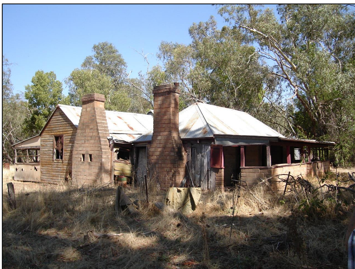
The old Warri homestead buildings in 2014
