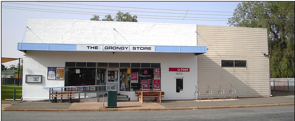
Above: The Grongy Store in November 2019.
