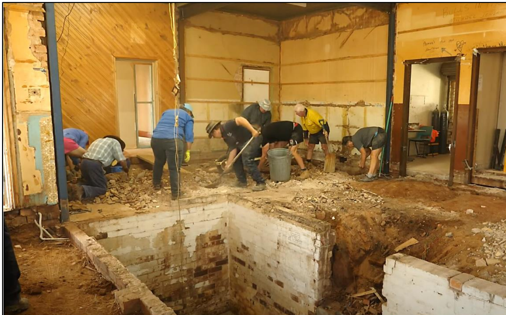
Left: The old cellar exposed during the renovations.
