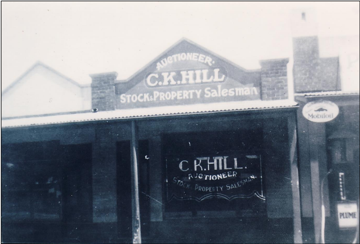
Above: CK Hill, auctioneers, to the south of Pomplun's garage, on allotment 10. Courtesy Ariah Park Community Project Committee.
