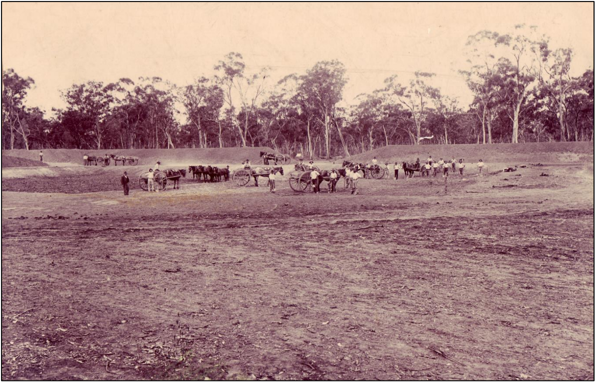
Above: Sinking the tank at Broken Dam. Courtesy Aria Park Community Project.
