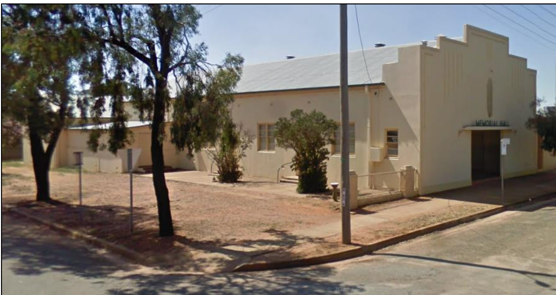
Above: The Memorial Hall in 2010. Courtesy Google Maps.
