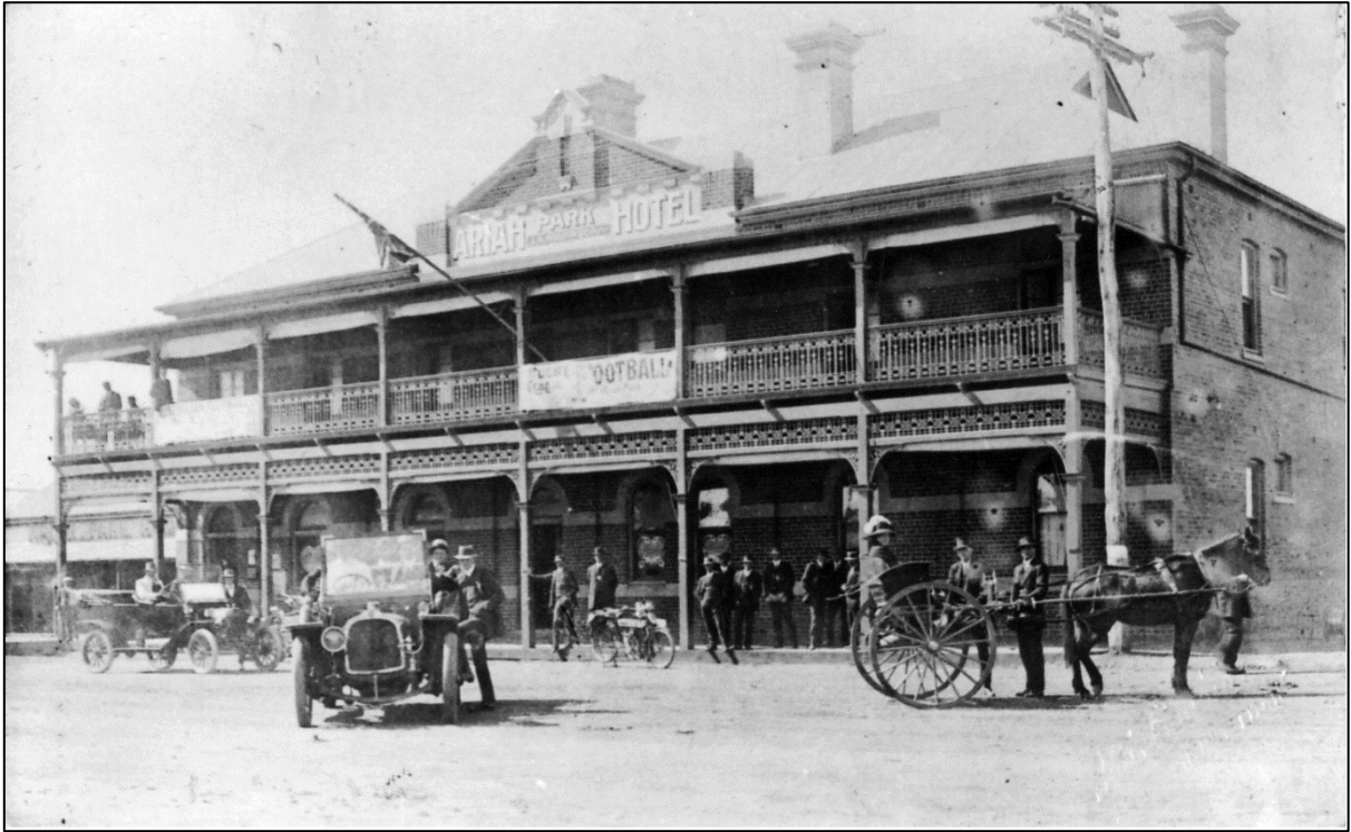
Above: The newer Ariah Park hotel with the old hotel just discernible, to the left.
