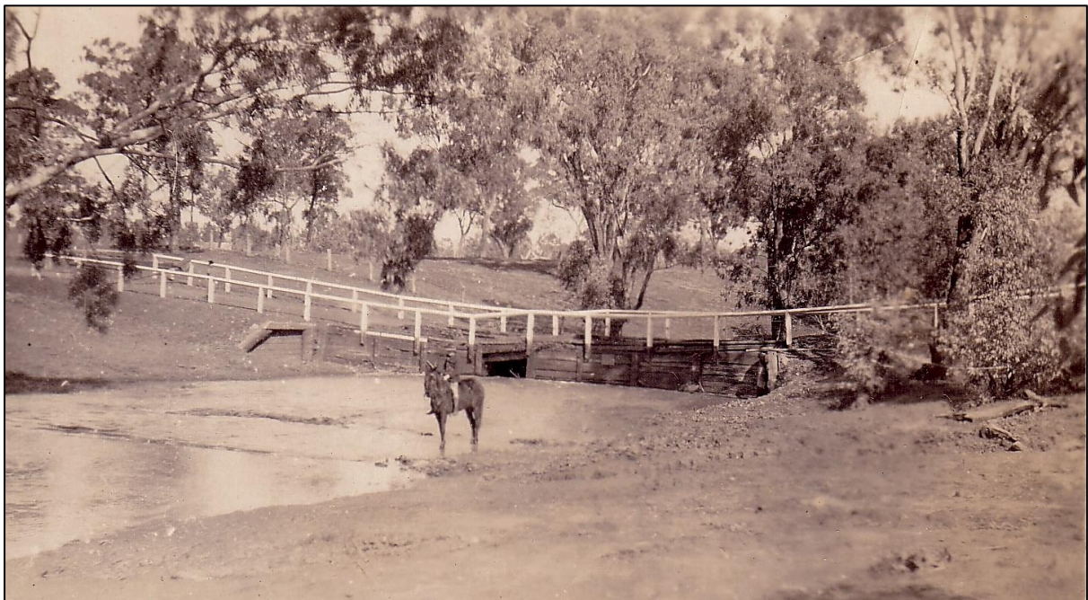
Above: Broken Dam bridge c.1916. Courtesy Ariaiah Park Community Project Committee.
