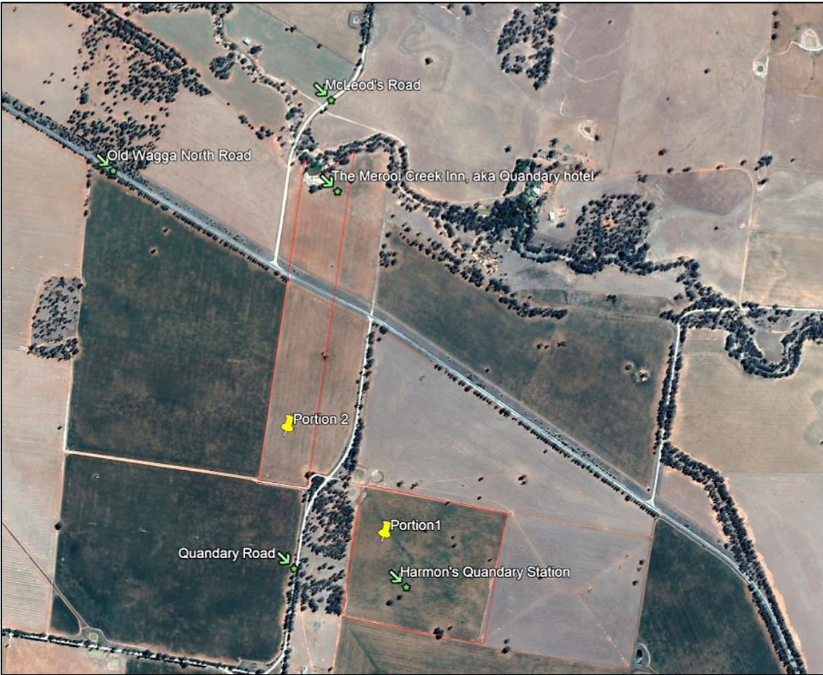
Above: A contemporary aerial view showing the locations of the Merool Creek Inn [aka Quandary Inn], and George Harmon's original Quandary Station block. Courtesy Google Earth.
