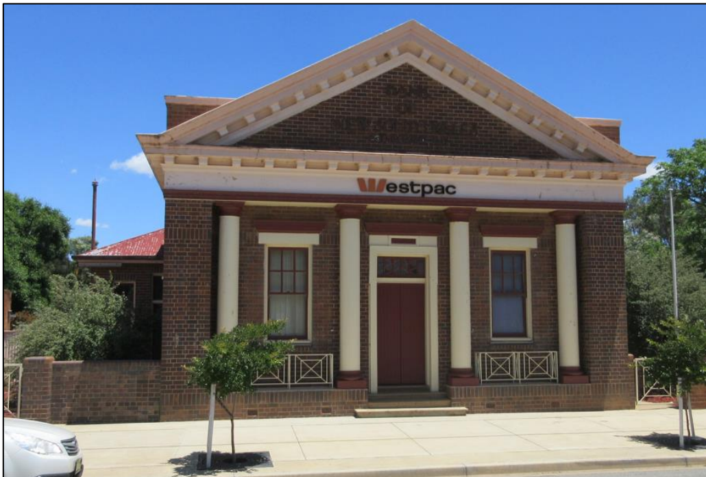
Above: Westpac Bank [former Bank of NSW building].
