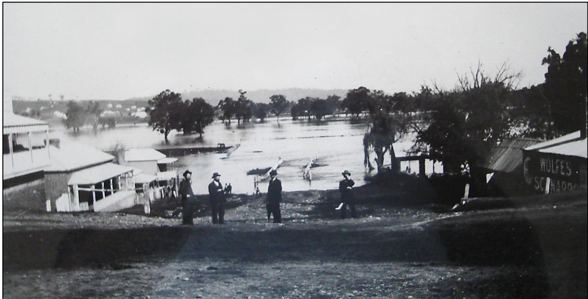
Above: Photograph of 1900 flood, taken from Sheridan Street, showing the extent of the area submerged during major flooding events. Courtesy Gundagai Museum.
