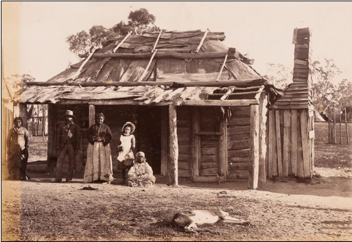
Above: An early house on Maloga Mission Station, c.1883. Courtesy State Library of Victoria. 26
