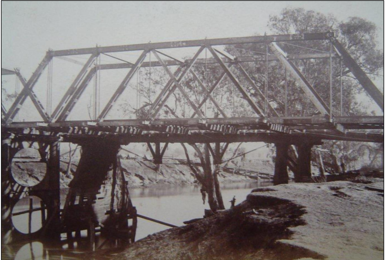
Above: Construction of the Hampden Bridge with the old Company Bridge still standing - on the downstream side. The old wharf can be seen in the background. Courtesy CSU Regional Archives.
