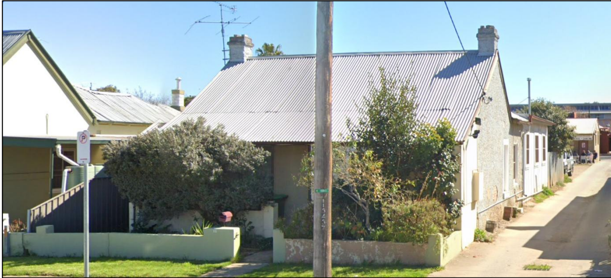
Above: 15 Cross Street. Courtesy Google Maps.
