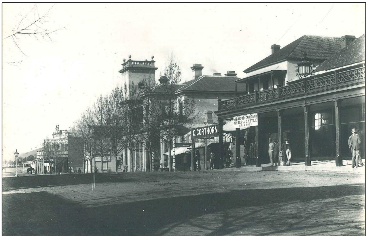
Above: Fitzmaurice Street west – from Australian hotel back to Union Bank.
