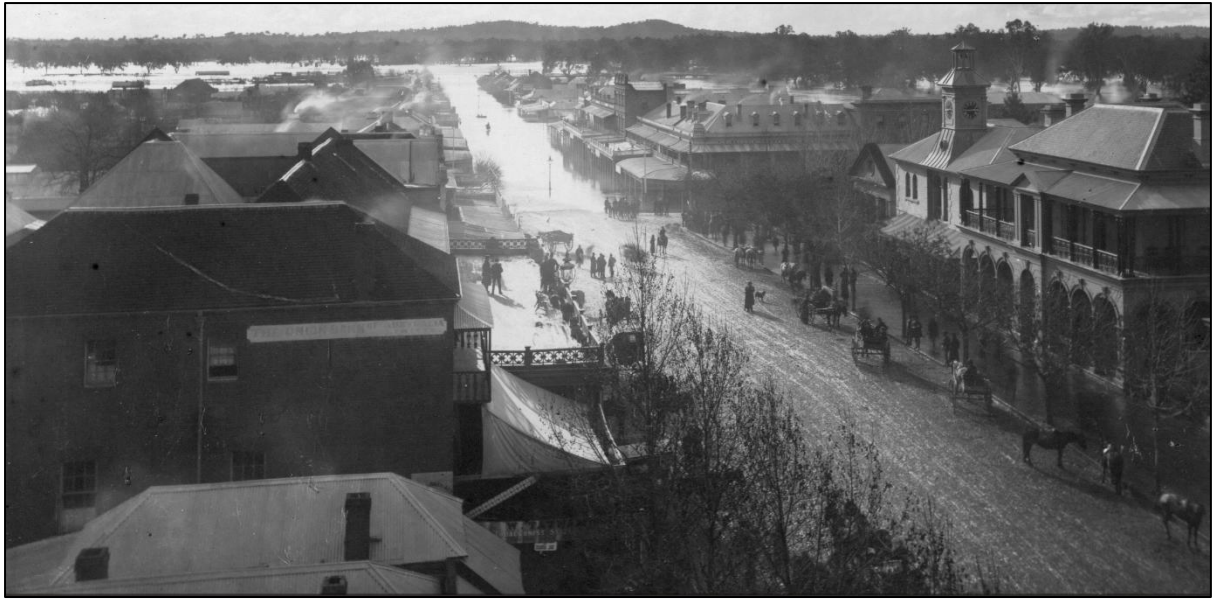
Above: Fitzmaurice Street view during major flooding [between 1876 and 1885]. The southern wall of the Australian hotel displays a sign reading "The Union Bank of Australia."
